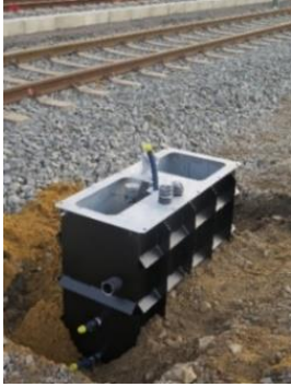
Image 3: The foundation console allows an easy installation of the TUnit.
